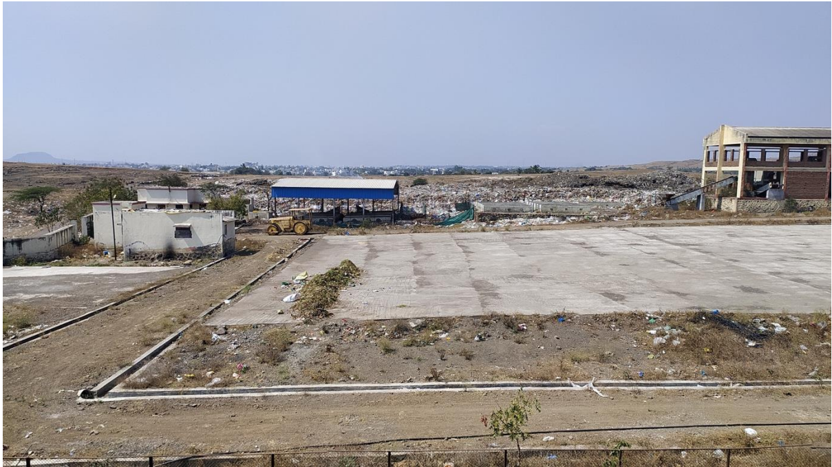
The implementation of SWM DPR is currently on-going in Sinnar. The slab (for windrow composting) and a shed for housing machinery are ready. Legacy waste in the behind the shed in the middle of the picture. Important to note that the ULB does not own the parcel of land where waste is currently dumped..
